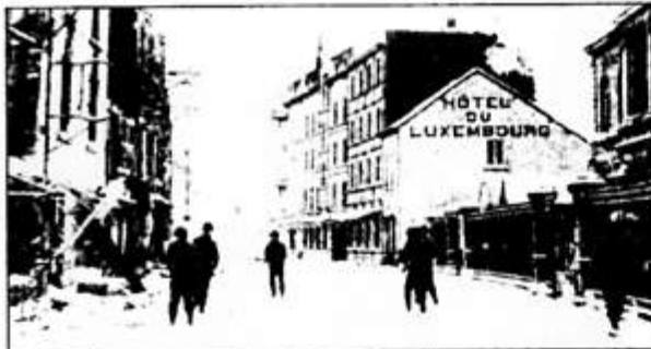
Then: Walking through war-torn La Roche in January 1945, US soldiers turn and pose in Rue Chamont [3] with the Hotel du Luxembourg in the background — though this is Belgium! Despite the snowy blanket covering the town, the destruction is self-evident.
