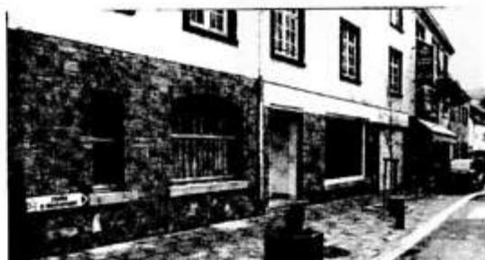
In spite of the restored buildings, the tank's resting place (2) can be pinpointed with complete accuracy — on top of the planter in the middle of this photo which stands outside the 1. et Vieille Auberge restaurant! The building on the left is No. 1 Villa Sassez; behind the author's position runs the Rue du Port heading to the northernmost bridge in Houffalize.
